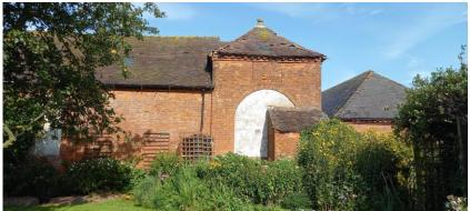
II as part of the Audleys Cross Farmhouse and ranges of farmbuildings. It is the right hand of the taller square corner sections with hipped roof which has suffered from the decay. Earlier surveys show that some sections including this were covered in ivy, which probably caused the decline of the mortar and the brickwork. This has been cleared but the decay now needs rectifying to halt the decay and repair the damage.
